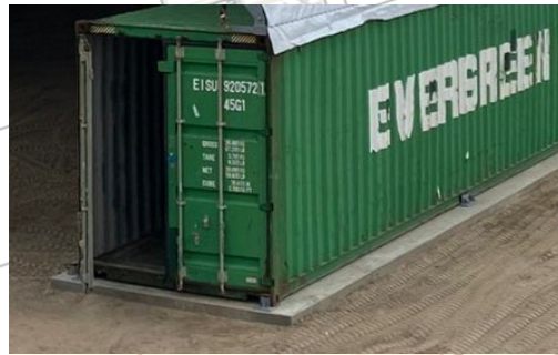
Full Concrete Pad with Base Plate Bracket Attachment
