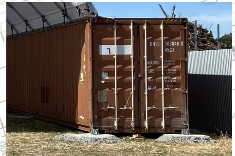
Concrete Pier Footing with Base Plate Bracket Attachment
