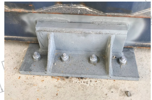
Base Plate Bracket #2 with Spacer (BP2S)
